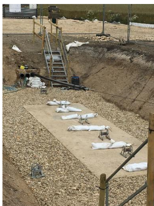
Figure 1.13 A: A typical jointing pit under construction. B. typical link box cover once backfilled (image courtesy of RWE Renewables)
